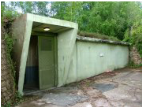
(Left) Aspidistra entrance tunnel
